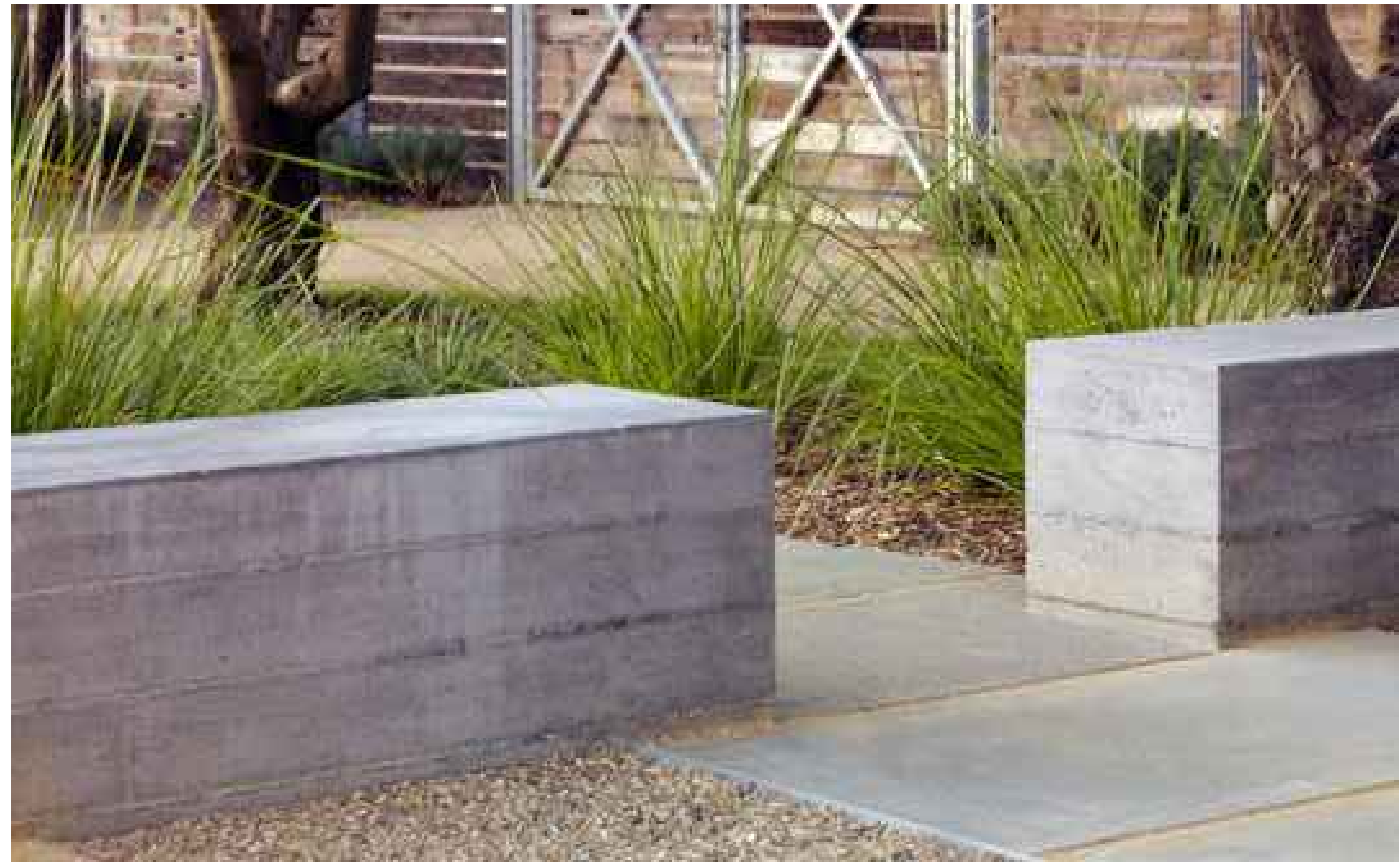
A CONCRETE SEATING w/DEFENSIVE ARM RESTS 4'oc +/- - FORMED IN-PLACE (18" ht x 18" wide x length varies)
