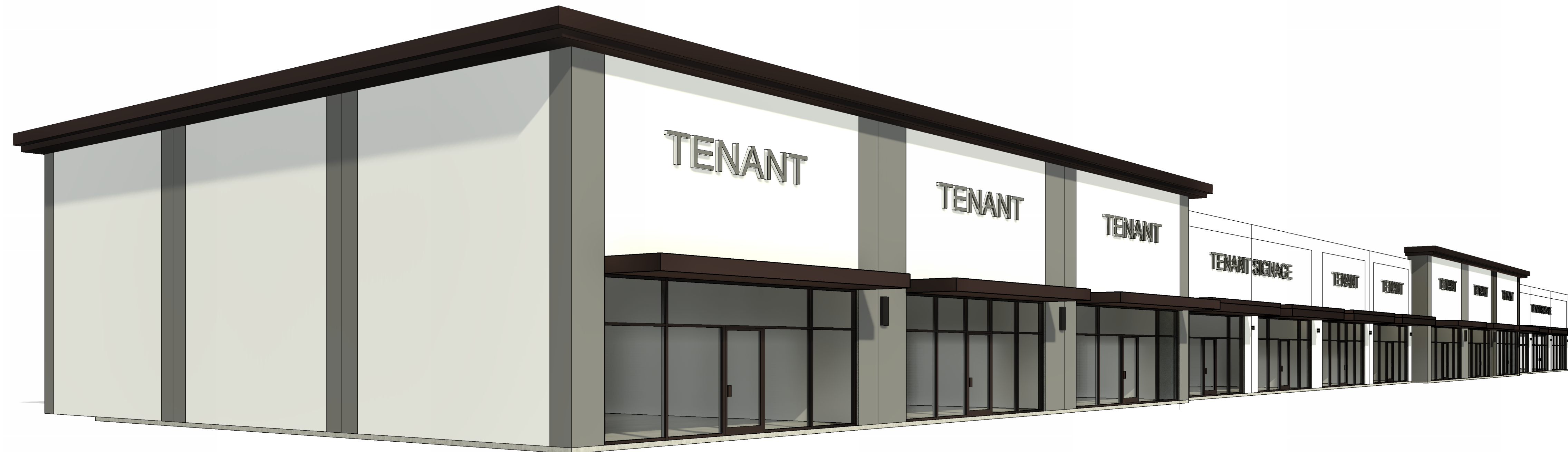
1 VIEW FROM NORTHEAST CORNER
